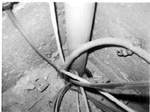
8250_GAINE TECHNIQUE Batiment H
