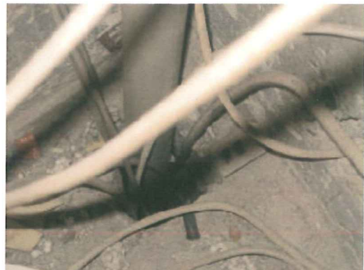
8267_GAINE TECHNIQUE Batiment C
