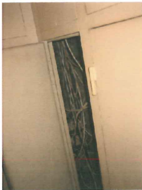
8248_GAINE TECHNIQUE Batiment H
