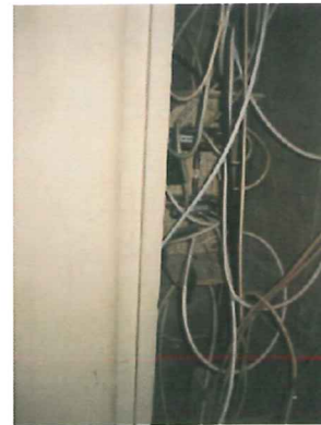
8249_GAINE TECHNIQUE Batiment H
